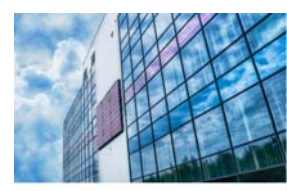
THE KEY TO A SUSTAINABLE BUILDING FAÇADE NL
